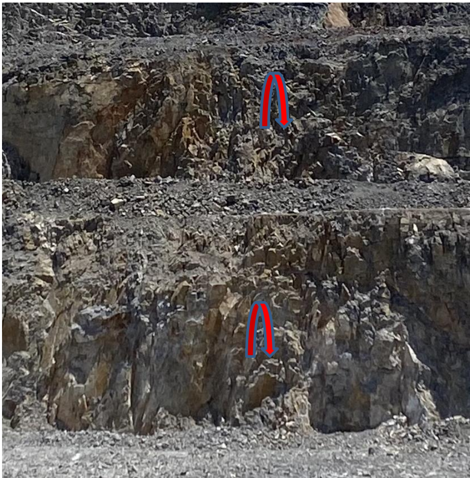
Figure 11. Example of toppling on the north wall of Pit 4 involving bench scale masses of rocks bounded to the rear by steep dipping joints from Set 3 having high persistences..
