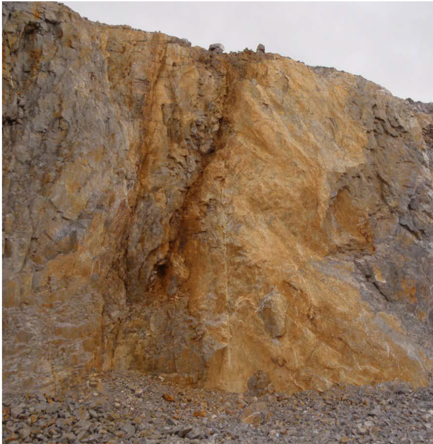
(a) Apertures within discontinuities daylighting in the north wall of Pit 4.
