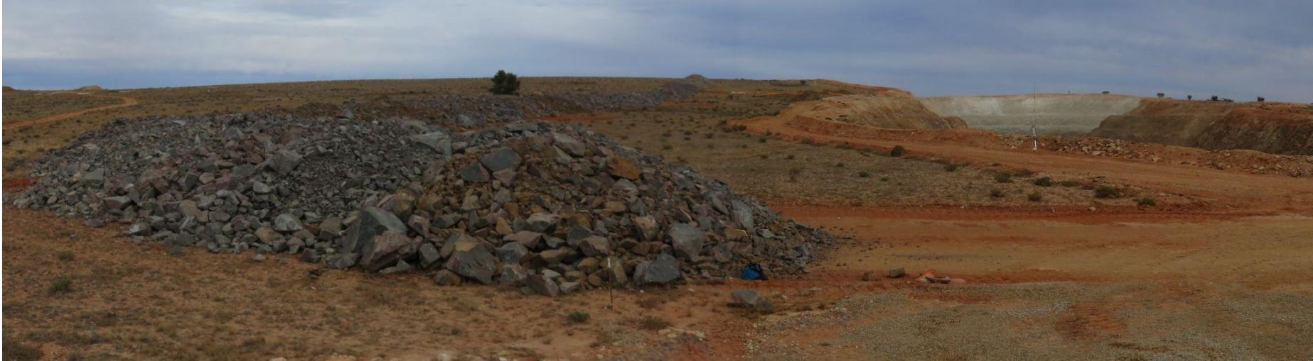
Figure 21. Example of an abandonment bund similar to those to be placed around Pits 2 and 3-4.
